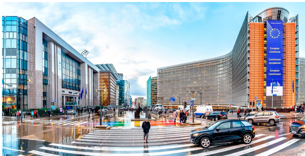
Panoramic view of the Berlaymont building, headquarters of the European Commission, in Brussels.
