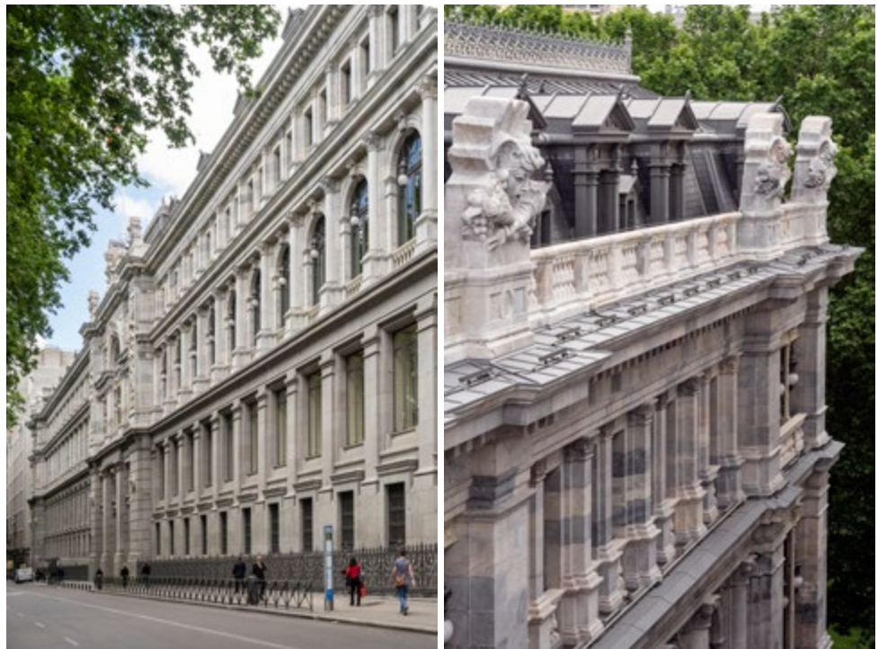
The façades on Paseo del Prado (left) and Calle Los Madrazo (right), seen from Cibeles, following completion of restoration and cleaning work. Main headquarters of the Banco de España.
